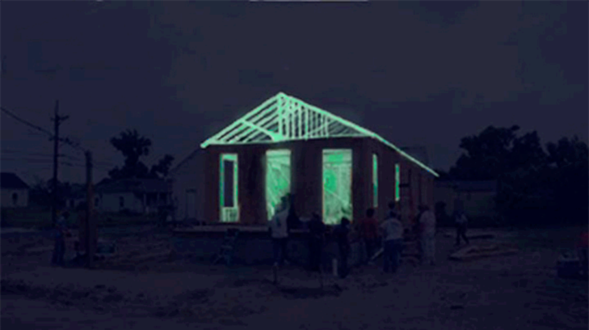
House under construction
